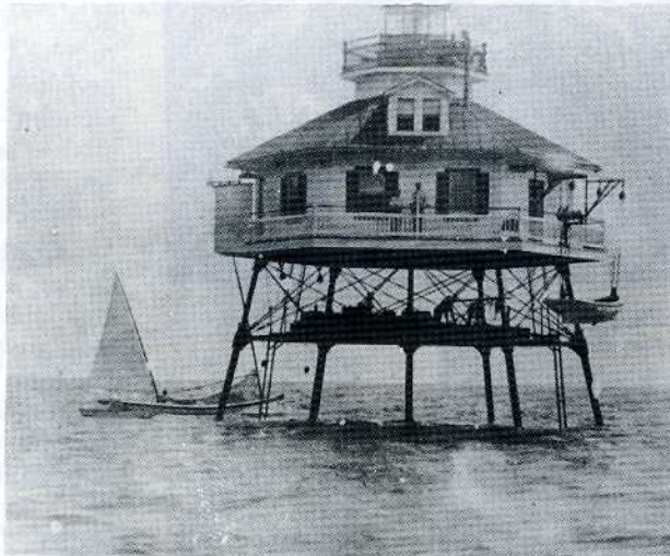
Drum Point Lighthouse, circa 1907. This early view of the lighthouse was thought to be nineteenth century, but recent evidence points to a later date. Just visible in the lantern is the narrow dark sector that warned mariners of the shoal off Sandy Point from 1899 to 1911. The platform underneath the lighthouse was probably not added until 1899. Keeper James Locke Weems may be the taller of the two men standing on the walkway. (Copied from a postcard owned by Mrs. Philip D. Lines)
