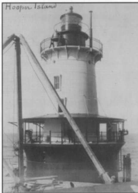
Hooper Island Lighthouse, shown shortly before completion in 1902. Photograph taken from the construction wharf with its wooden derrick prominent in the foreground.
