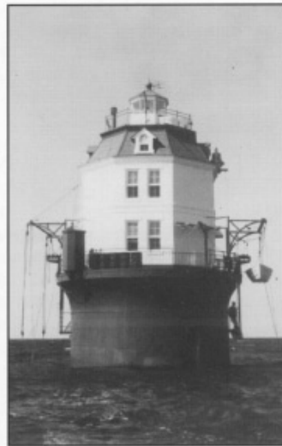
Point No Point Lighthouse before automation.
